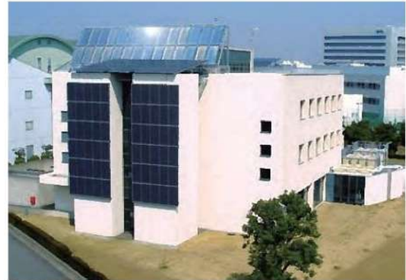
The building with which Japan's first ZEB was achieved through renovation. We installed PV panels and solar collectors.
