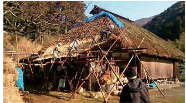
Rethatched roof of a traditional folk house in Yamaguchi prefecture
