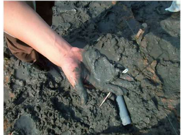
Deteriorated lime-treated clay in a marine environment
