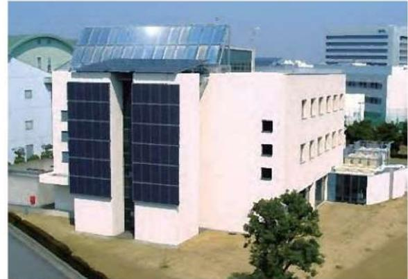
The building with which Japan's first ZEB was achieved through renovation. We installed PV panels and solar collectors.
